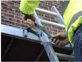
Fig 1 Easi-Dec Ladder spurs.
