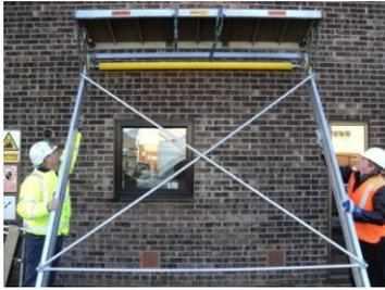
With bent Legs and a straight back, lift the Window-Dec firstly to waist height, then using your arms to offer it to the wall and roll it up into position.
