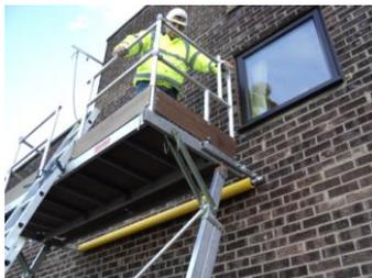
Climb onto the Platform and position the rear Uprights into the rear locating sockets on the platform for both the Left and right handed Guardrail.
