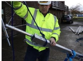
The Hoisting Assembly needs to be secured before lifting, using the supplied Assembly Straps as illustrated. Then tie rope around the top part of the frame ensuring it is properly secure ready for lifting.
