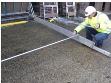
Fit the Horizontal Brace over the retaining studs.
