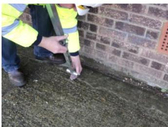
Drop the feet to the ground and take it up to the next hole and secure with the Pin and 'R' Clip. Ideally a finger's clearance under them to ensure the Window-Dec Platform remains in contact with the wall.
