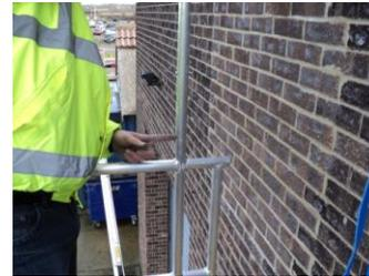
Make sure the support tubes are completely flush with the gate to ensure full connection. **REMEMBER: Raise the toe-board across the Ladder access point before using the Hoist.**
