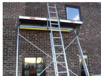
The Ladder is placed against the Platform, extended 1 metre above Platform level between the Ladder Restraints of the Platform and sided to the right to allow enough room to step through on the left hand side.
