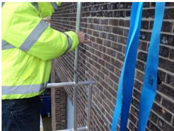
Lift the whole assembly by holding the support tubes and then position these tubes over the Hole in the Guard rail posts. **NOTE:** Two operatives are required to complete the assembly.
