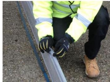
Pull out the clips and release the two Braces from their stowed position.
