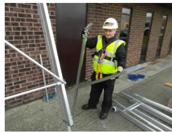
Fit the Back Legs by removing the Middle Pin first, holding onto it and lowering the brace.
