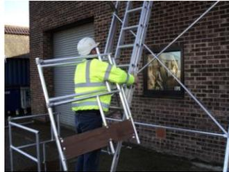
Position the Right Guardrail over your shoulder, when climbing the Ladder, maintain three points of contact. **REMEMBER:** When fitting the Guardrail to the Left hand side of the Platform carry up on the Left shoulder.
